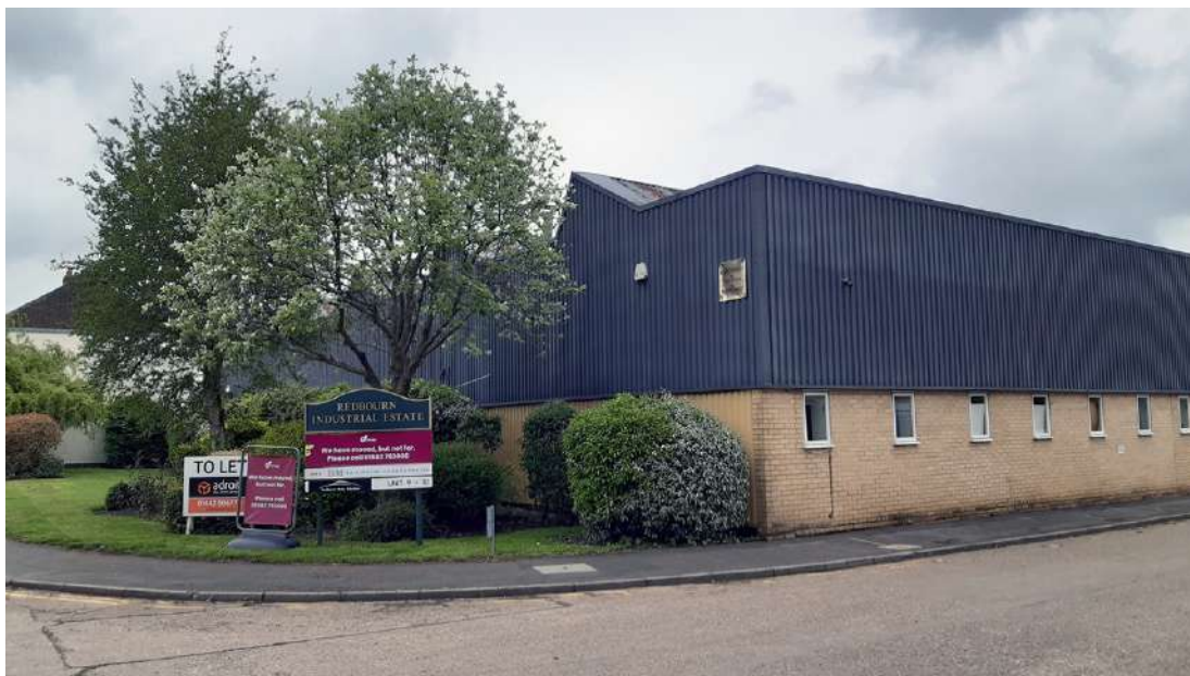
Figure 24: Redbourn Industrial Estate
