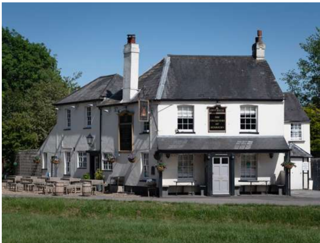
Figure 35: The Cricketer’s Pub, Redbourn – a Locally Listed Building
