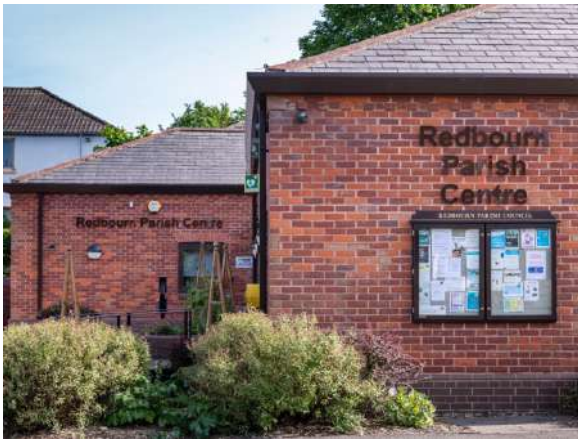
Figure 7: Redbourn Parish Centre
